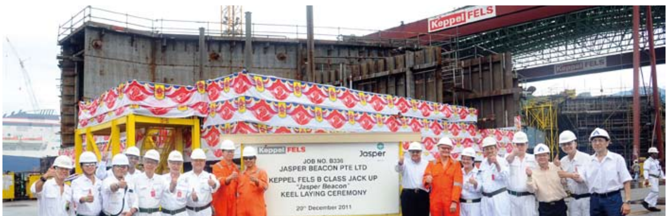
Construction on the KFELS B Class jackup rig, Jasper Beacon, has followed closely on the heels of its sister rig, the Jasper Adventurer
